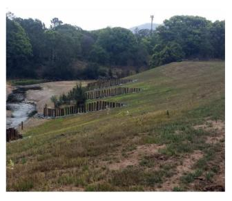
**Before and After Photos** - January 2019 sheer banks and September 2019 bank re-profiled and pile fields and rock armouring to slow flood waters. Native trees and shrubs planted to further stabilise the bank.
