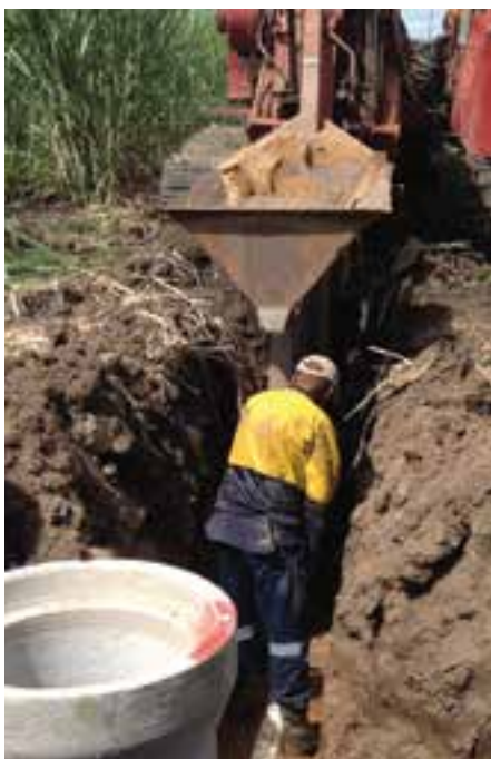
PICTURED: Installation of sub-surface drainage to allow leaching to commence.
