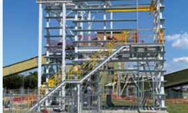
Steel framing underway for the Transfer Tower #1 at the CUI Project at the Bundaberg BST.
