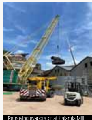
Removing evaporator at Kalamia Mill
